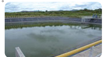
Bridgestone Carbon Black (Thailand) Co., Ltd.(BSCB)の雨水貯留池
